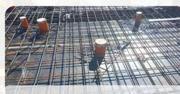
INSTALLATION OF PIPE SLEEVES
