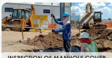
INSPECTION OF MANHOLE COVER
