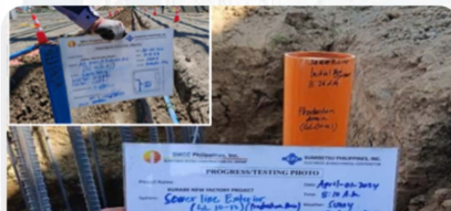
GRAVITY TEST ON AC DRAIN AND SEWERLINE
